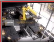
Picking to Conveyor
